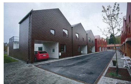
Buildings in direct contact with the street (shown Äppelträdgården, White Architects).
