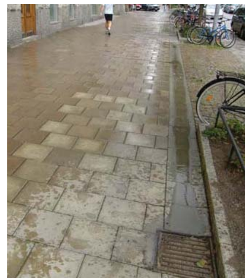
Images from Stockholm City of water being channelled to planting beds
