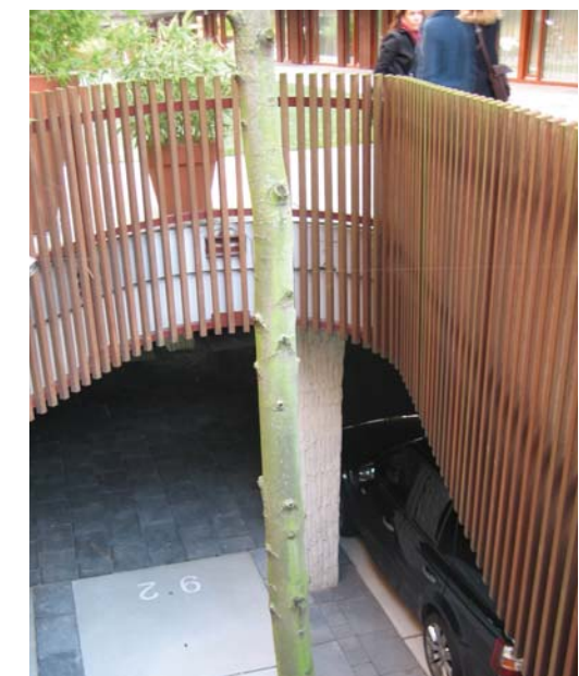
Using planting as a vertical element to define the interface between a half-basement carpark and raised courtyard.
