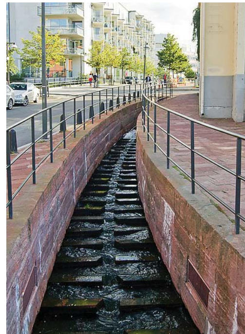
Stormwater aeration channels can act as attractive design features (shown: Hammarby sjöstad, Stockholm)
