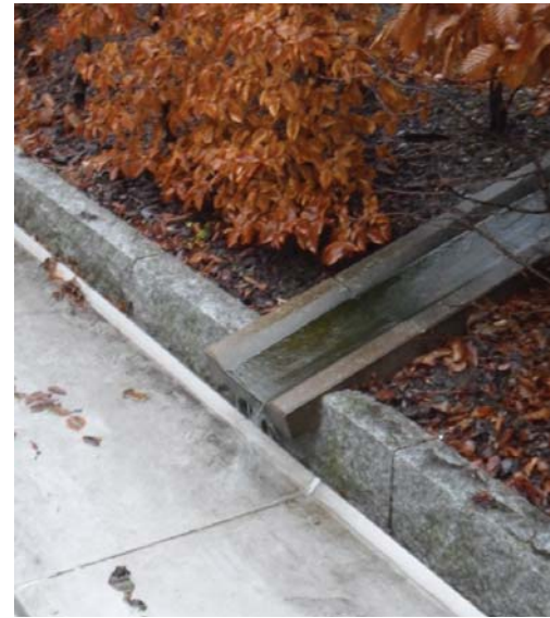
Hammarby Sjöstad integrated water channels leading stormwater from roof tops to the street network
