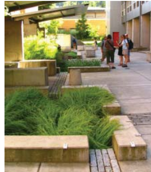
'Flow Through' rain garden which uses plant material to take up pollutants while preventing infiltration into the groundwater.
