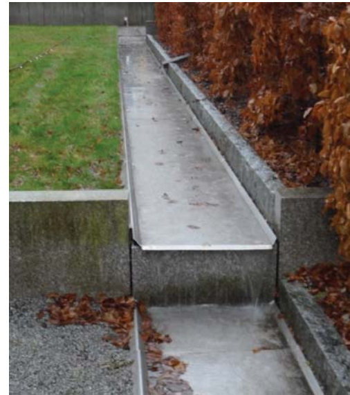
Hammarby Sjöstad integrated water channels leading stormwater further afield.
