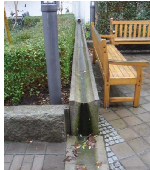
Hammarby Sjöstad integrated water channels leading stormwater from roof tops to the street network
