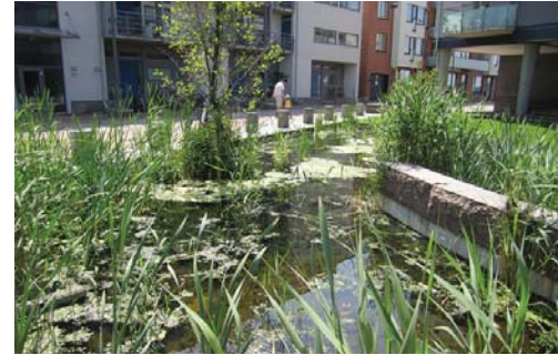
Rain gardens make stormwater visible after periods of rain (shown: Västra Hamnen, Malmö).
